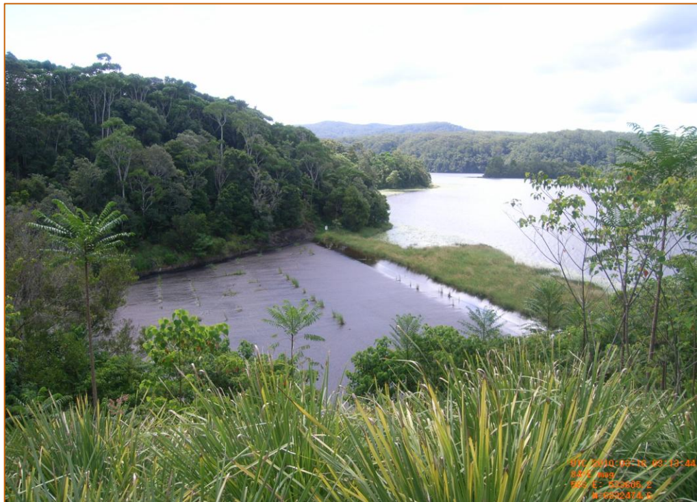
Plate 16: Rocky Creek Dam spillway showing vegetation in between the high water and mean water mark
