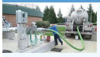
FOGs are energy rich organic material with three-times higher potential for CH<sub>4</sub> generation than sewage sludge. When co-digested with sewage, the addition of FOG as a feedstock benefits generation of biogas in anaerobic digestion and assists the WWTP to reach energy neutrality in addition to additional revenue from the gate fee for FOG disposal.
